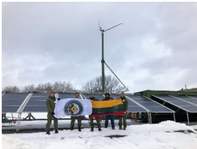
Figure 19. December 2018 - April 2019: Test in extreme temperature, requested by Canadian Government.
